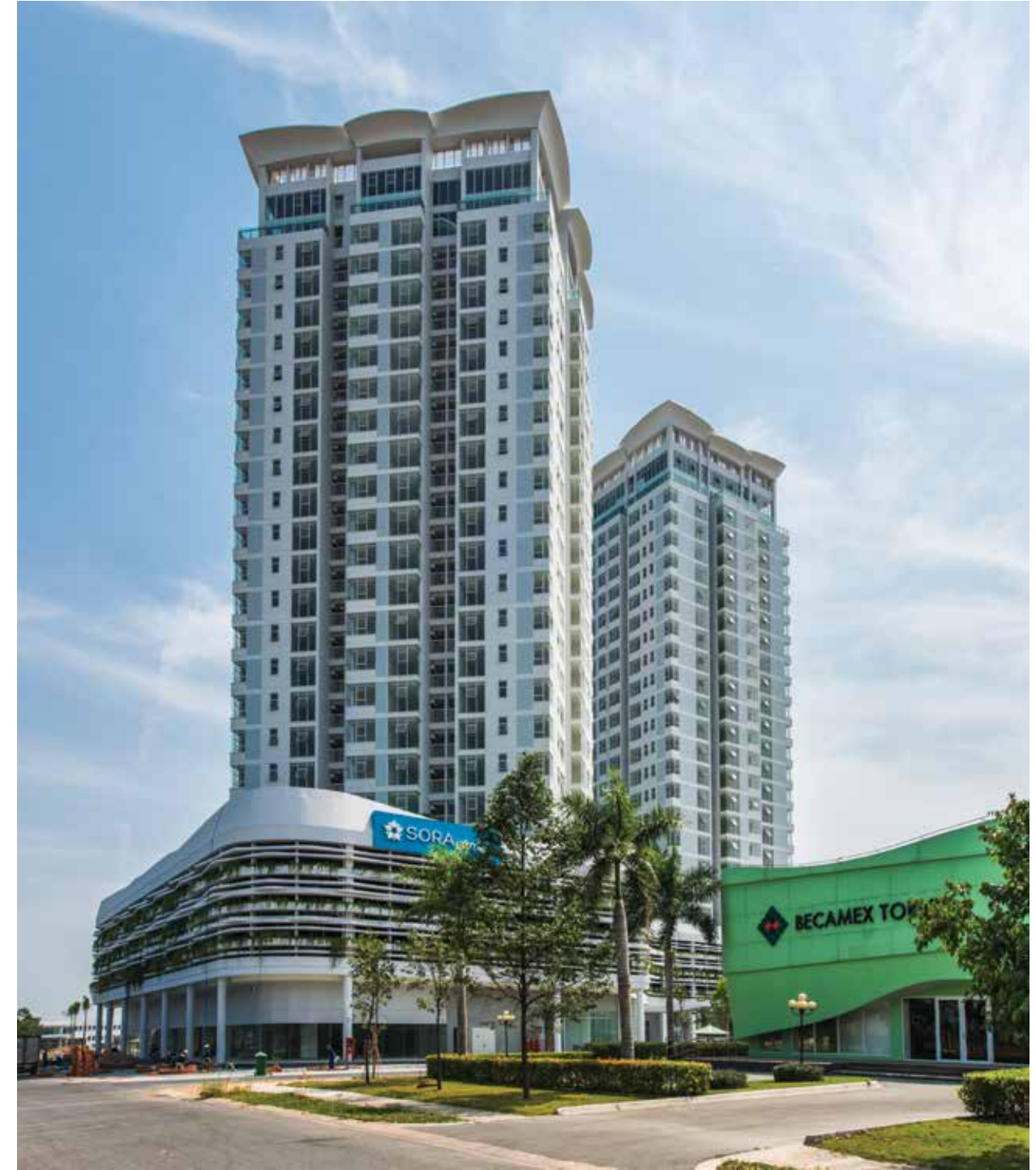
SORA GARDENS 1 Main Contractor
